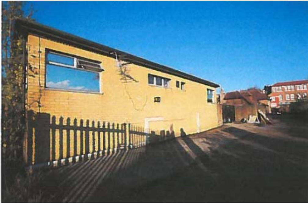
Front of the site
